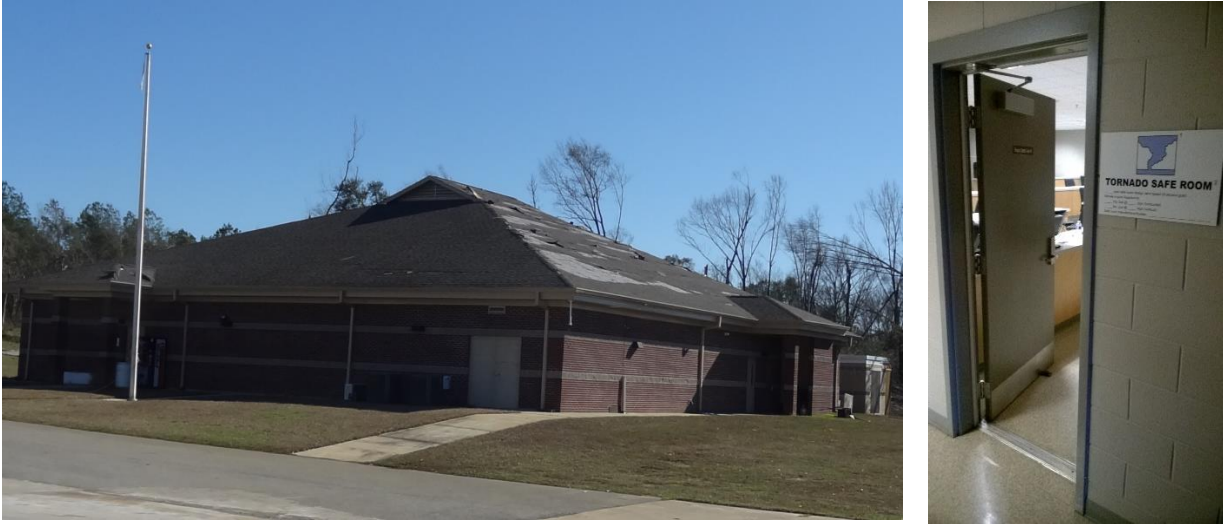
Figure 19: Training center (left) and tornado safe room within the building constructed out of reinforced CMU block with ICC approved doors and no windows (right).
