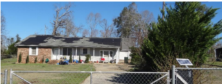
Figure 12: Some roofs had asphalt shingle roofing removed (near edge of tornado path (Source: UF WHDAG))
