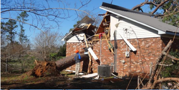
Figure 10: Uprooted pine tree cuts through a light-framed wood residential structure (Source: UF WHDAG)
