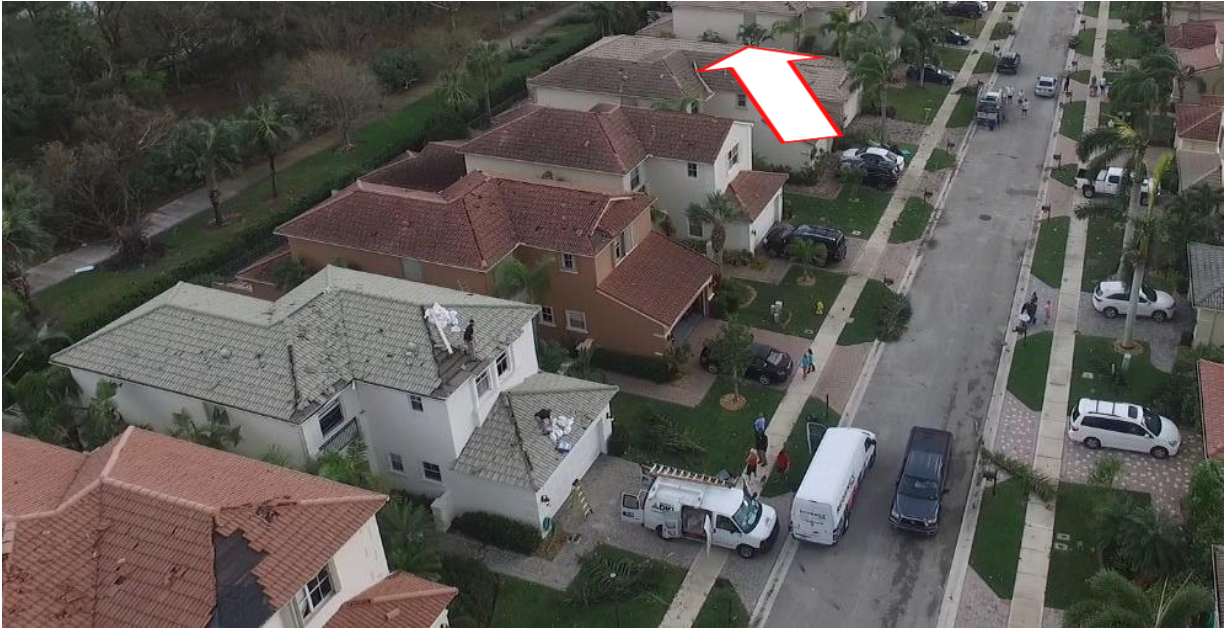
Figure 30: Clay tile failure on multiple roofs in Palm Beach Gardens from the EF1 tornado. The approximate direction of tornado travel is indicated by the red/white arrow. Photo by Michael Buczyner .
