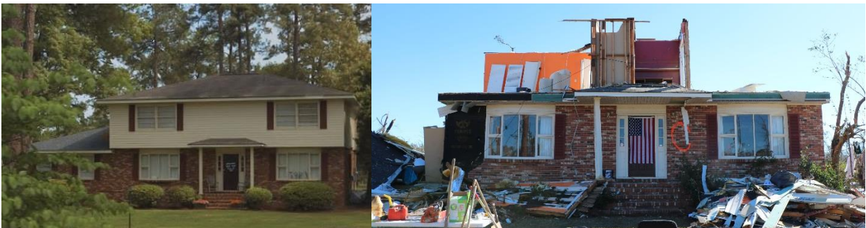
Figure 17: (Left) Before: Google Streetview; (Right) After: Second floor destroyed, few interior walls remaining (Source: UIUC)
