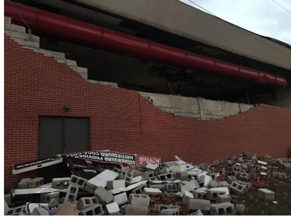
Figure 24: Damage to institutional buildings at William Carey University (Left: @ WmCareyU ; Right: @ RyanMooreMS ). Note the lack of grout in-fill in a large section of the CMU wall, which crumbled under the wind loads as a result.
