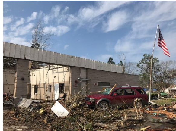
Figure 25: Damage in Hattiesburg to an apartment complex (left, by Ryan Moore ) and to Fire Station 2 (right, by Ryan Moore ). The large openings shown in the fire station allow wind to pressurize the interior space, enhancing wind loads on the roof system.
