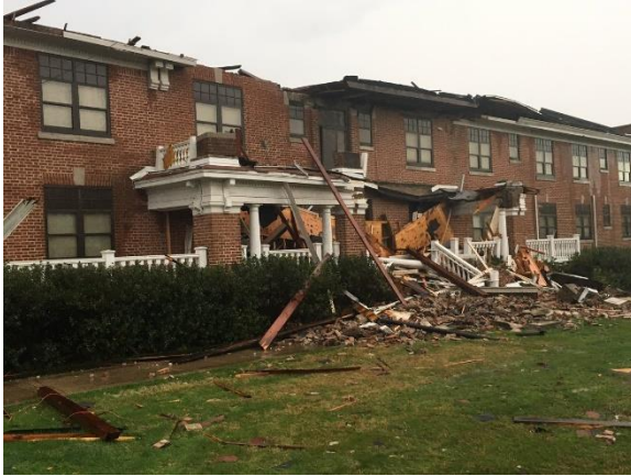
Figure 24: Damage to institutional buildings at William Carey University (Left: @ WmCareyU ; Right: @ RyanMooreMS ). Note the lack of grout in-fill in a large section of the CMU wall, which crumbled under the wind loads as a result.
