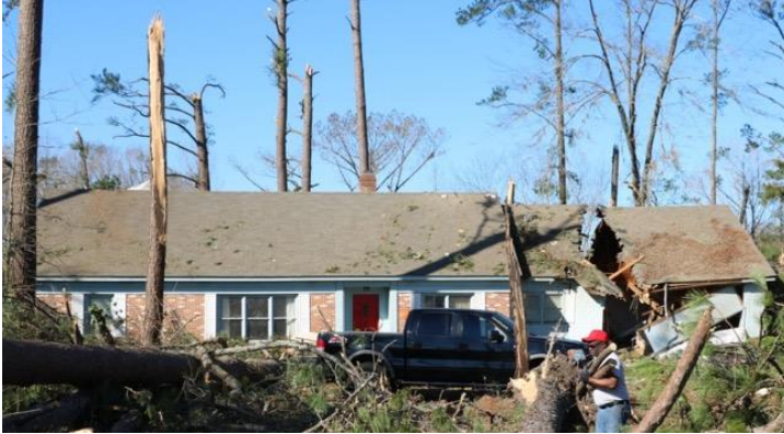
Figure 11: Light-framed wood gable roof structure located near north edge of tornado damaged by fallen tree. Only superficial damage elsewhere on structure (Source: UIUC)
