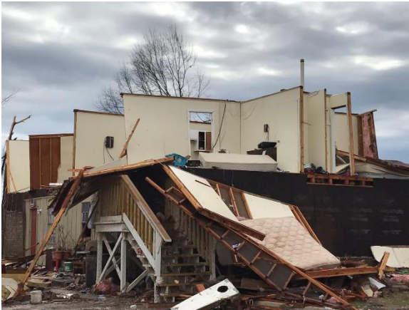
Figure 25: Damage in Hattiesburg to an apartment complex (left, by Ryan Moore ) and to Fire Station 2 (right, by Ryan Moore ). The large openings shown in the fire station allow wind to pressurize the interior space, enhancing wind loads on the roof system.
