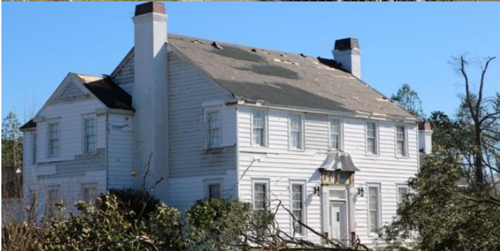
Figure 13: A 2-story structure in "Neighborhood 1" suffered asphalt shingle and siding without any obvious structural damage (Source: UIUC)
