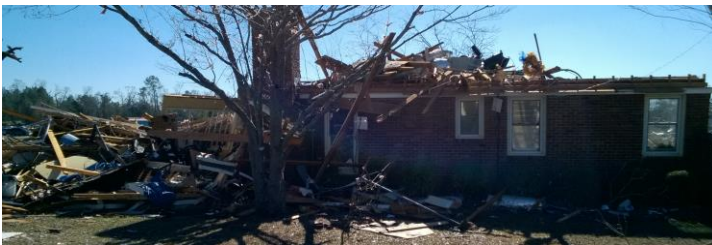
Figure 16: House located on the Sylvester Rd, adjacent to Albany Baptist Church lost its roof and several exterior walls collapsed (Source: UF WHDAG)
