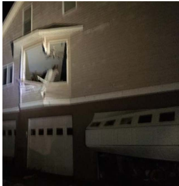
Figure 6: Bay window breached and garage door blown out in home along Old Pond Rd. Photo courtesy of Stephanie Maxwell, WSOC Channel 9
