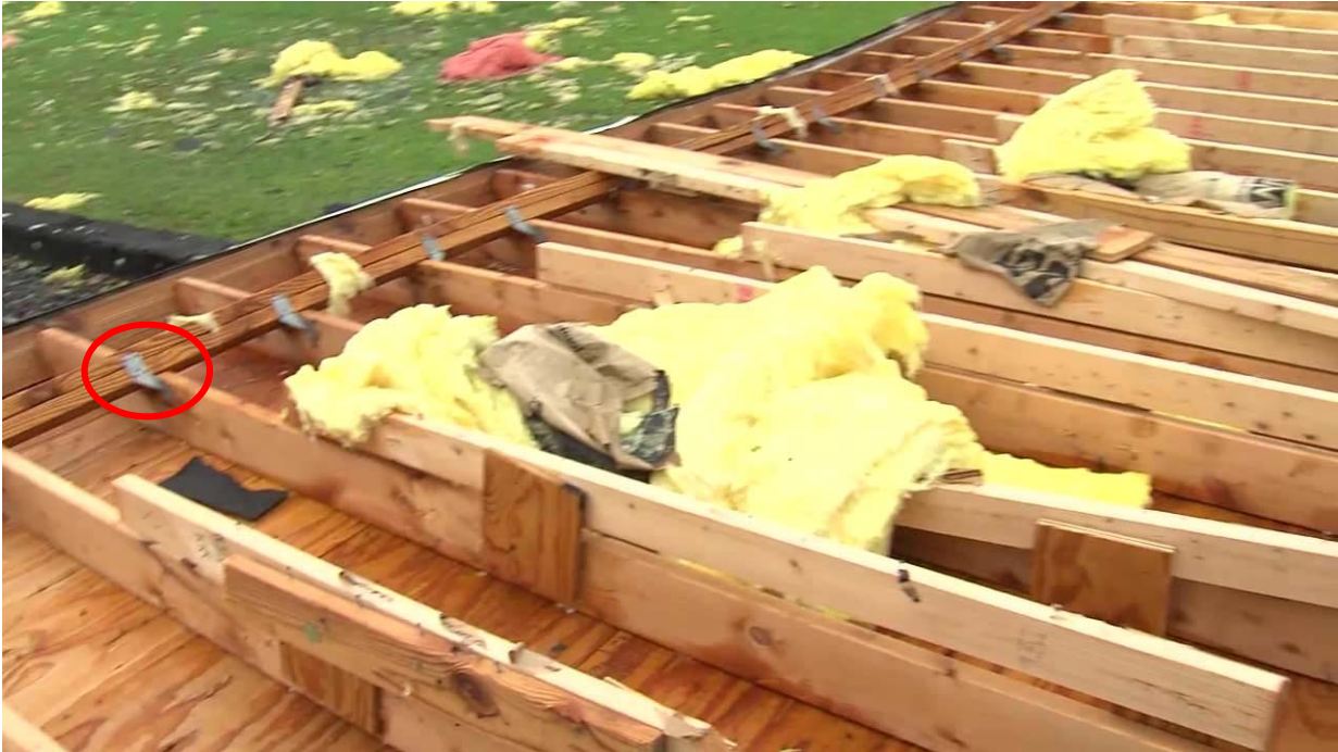
Figure 10: Hurricane straps present between rafters and wall top plate. However, the wall top plate separated cleanly from the wall structure and failed along with the roof, indicating the load path between the wall plate and vertical studs may have been the critical failure point resulting in the observed damage to this home (Photo courtesy of ABCNews4.com ).
