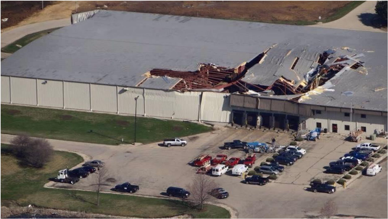
(a) Aerial view of damage to the main Crest Foods Warehouse in Ashton, IL ( Courtesy Joe Gomez ). The roof above the west loading docks collapsed.
