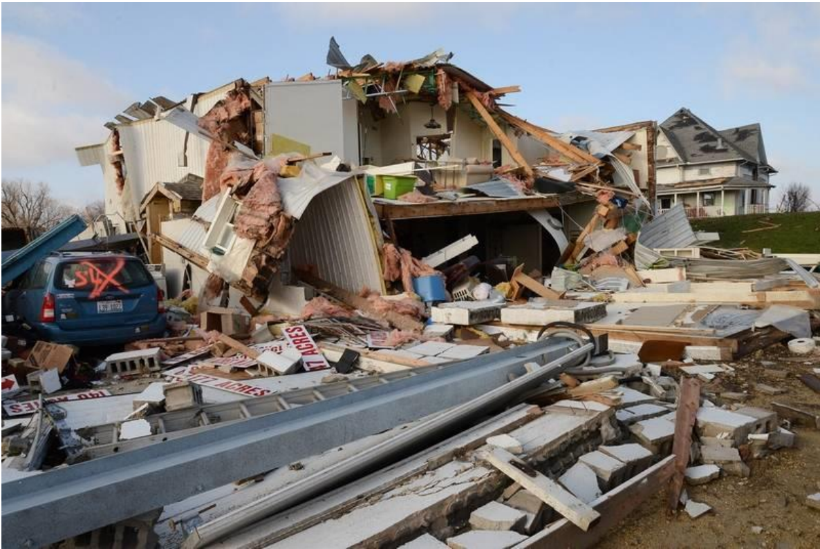
Figure 11: Damage to a wood-frame home in Fairdale, IL.
