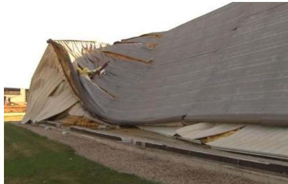
(c) Collapsed Walls and Roof, possibly in the mixing facility.
