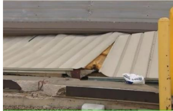
(e) Partially exposed foundation
