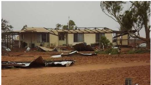
Figure 14. Roof loss at batten-to-truss connection in Carnarvon (Courtesy: Mary Bettini)
