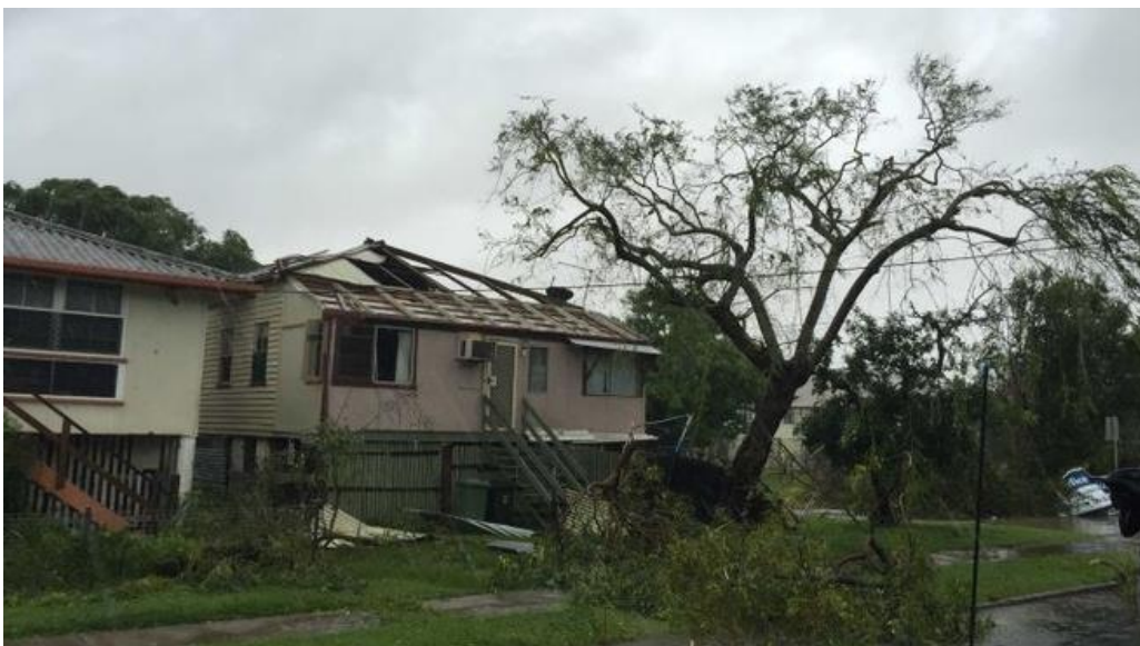
Figure 9. Batten and cladding damage in Yeppoon (pre-1960's house) (ABC News)
