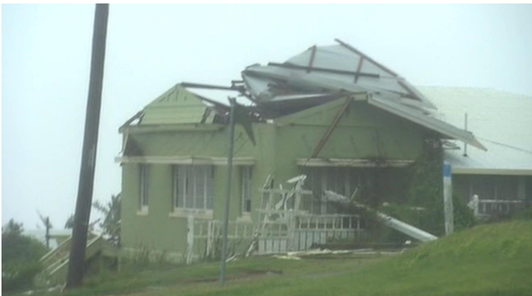
Figure 11. Roof damage to a home in Yeppoon caused by Tropical Cyclone Marcia. Photo courtesy of 7News Brisbane.
