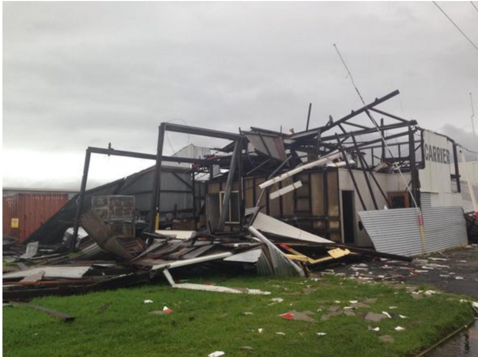
Figure 16. Structural damage to local business in Rockhampton. Courtesy Louisa Rebgetz .
