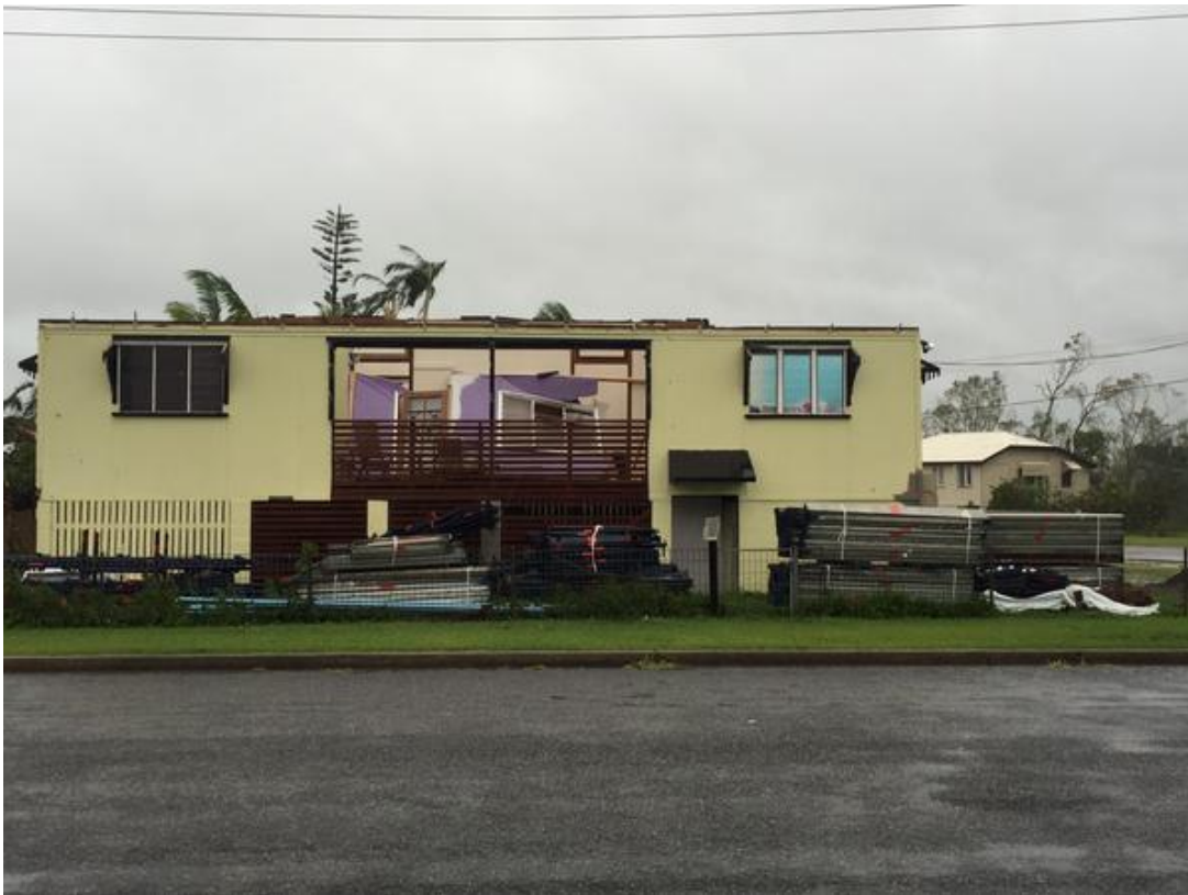
Figure 10. Fibro house (est. pre-1970's) with missing roof in Yeppoon (ABC News)
