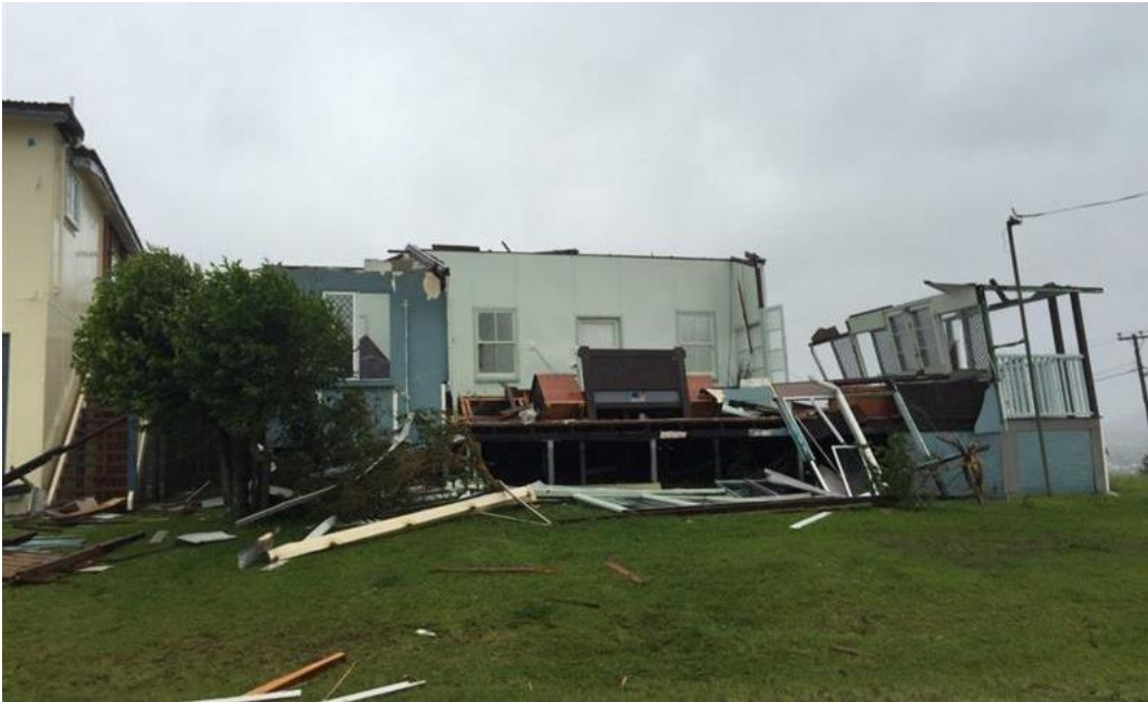
Figure 12. Roof removed and exterior walls collapsed in a home in Yeppoon. (ABC News)
