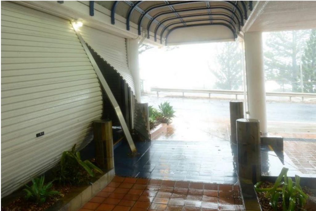
Figure 8. Roller doors blown outward at Yeppoon Hotel (Google Images)
