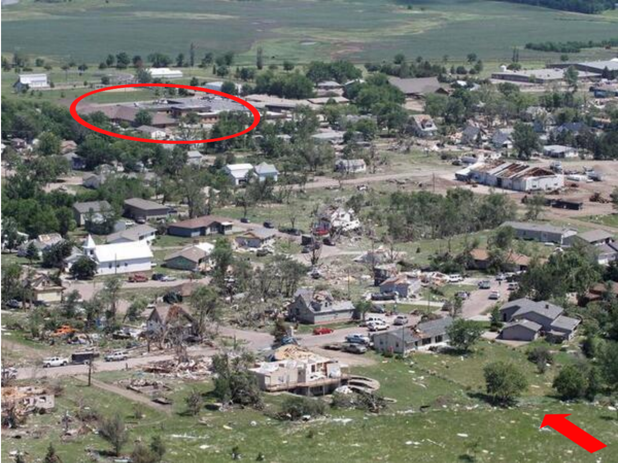
Figure 10: Aerial view of the EF-2 damage in Wessington Springs, SD from a tornado on June 18, 2014. The red arrow indicates North in this view. The red oval gives the location of Wessington Springs High School, which narrowly avoided a direct hit. (Source: Argus Leader.com )
