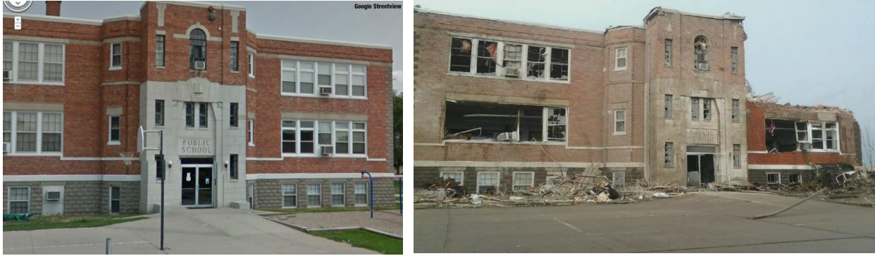
(e) Pilger Middle School ( before ) looking N (f) Pilger Middle School ( after ) looking N
