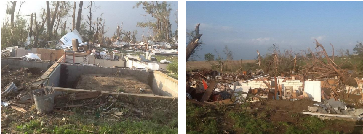
Figure 5: EF-4 damage 4 miles SSE of Wakefield, NE to two homes built in the early 1900's. (Source: NWS Toolkit, Omaha Office)
