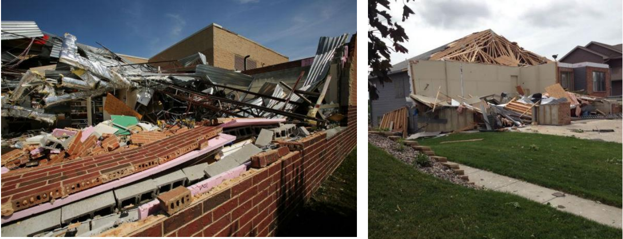
Figure 9: Collapse of classroom wall at County View Elementary school (left) and wall and roof failure at a nearby home (right) (Source: Wisconsin State Journal ).
