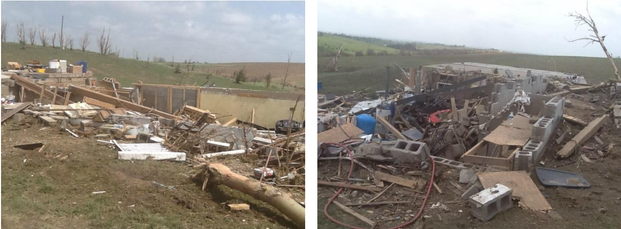
Figure 4: EF-4 damage (left) and EF-3 damage (right) 5 miles north of Stanton, NE (Source: NWS Toolkit, Omaha Office)
