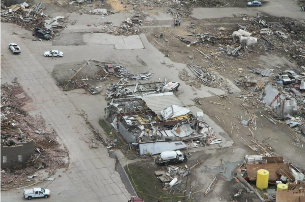
Figure 17: Looking east at damage to Farmer's Co-op in Pilger, NE after EF-4 tornado (Source: NEMA )
