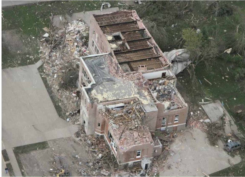
Figure 16: Aerial view of Severe Damage to Pilger Middle School (Source: NEMA )
