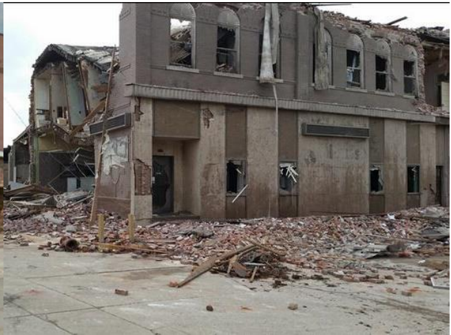
(b) Midwest Bank (after) looking NW
