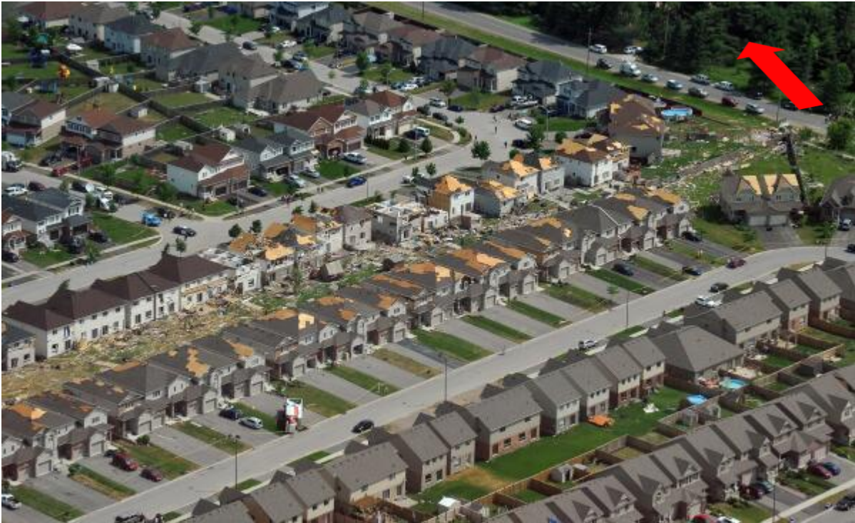
Figure 6: Aerial view of damage to Angus, Ontario from EF-2 tornado. North is approximately indicated by the red arrow. (Photo Courtesy of Ian McInroy)
