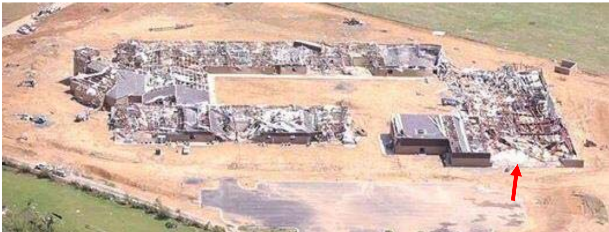
Figure 14. Severe damage to new Intermediate School in Vilonia, AR set to be opened Fall 2014. Red arrow indicated location and direction of photo shown in Figure 15.
