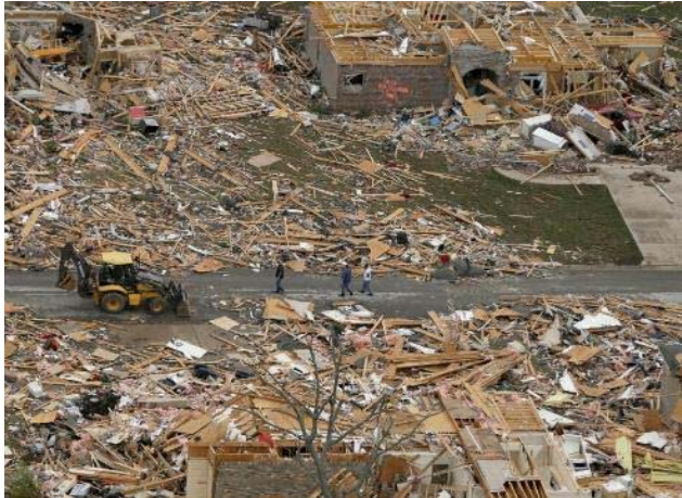
Figure 9. Severe damage in the River Plantation development east of Mayflower, AR
