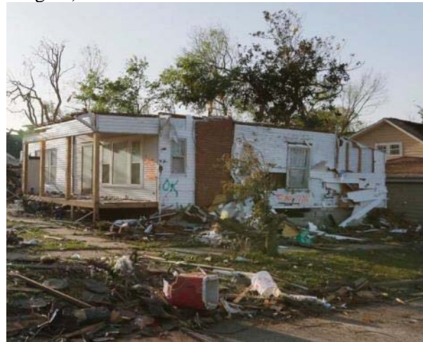
Figure 7. Degree of Damage 6 (104 mph - 142 mph). Possibly an EF2 rating. (AP Photo/Orlin Wagner)
