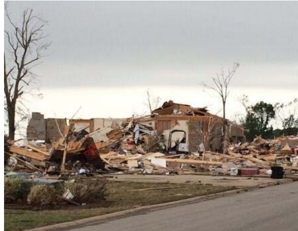
Figure 10. Roof destroyed from home in River Plantation development
