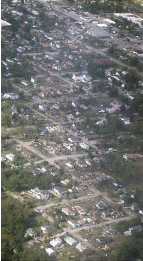
Figure 5. Aerial view of damage through Baxter Springs, KS (AP Photo/Orlin Wagner)
