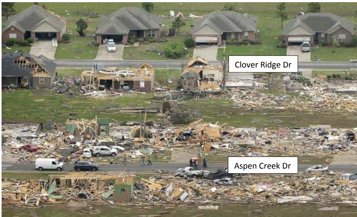
Figure 18. Looking North over the development after the tornado. Note the gradation of damage present with the garage doors collapsed outward along the north side of Clover Ridge Dr. (Photo Courtesy of USA Today)
