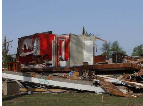
Figure 6. Degree of Damage 7 (113 mph - 153 mph). Possibly an EF2 rating. (AP Photo/Orlin Wagner)
