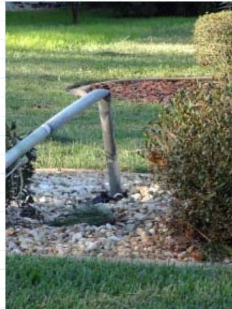
Figure A-2: Flag pole buckled at base. Note that portion of pole below ground has been pulled out of ground
