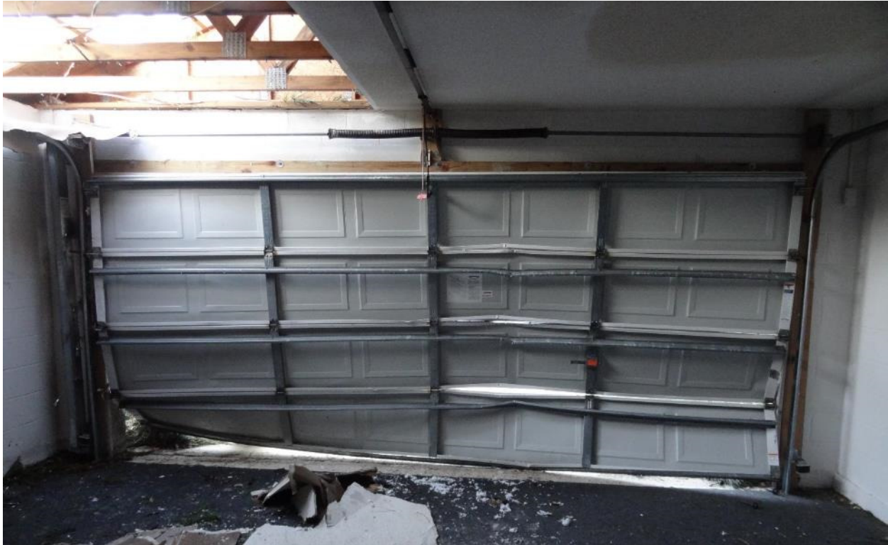
Figure B-1: Buckled garage door at 30 Barring Pl
