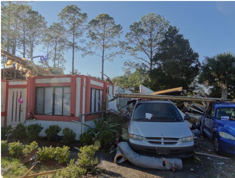
Figure 11: Removal of large portions of roof and collapse of walls to 1988 home with significant termite damage
