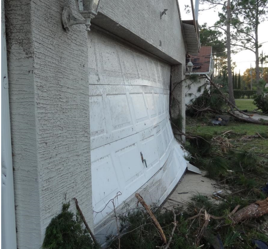
Figure B-4: View of buckled garage door from outside
