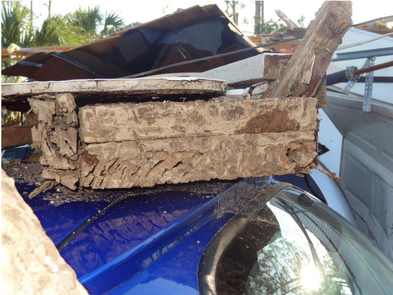
Figure 12: Termite damage to structural wood header over garage door opening.
