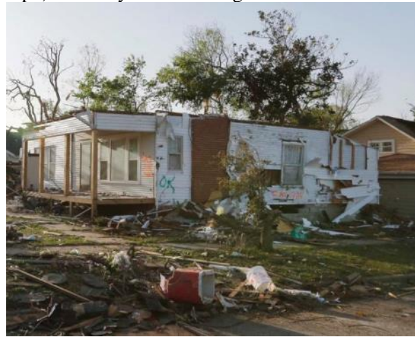
Figure 7. Degree of Damage 6 (104 mph – 142 mph). Possibly an EF2 rating.
