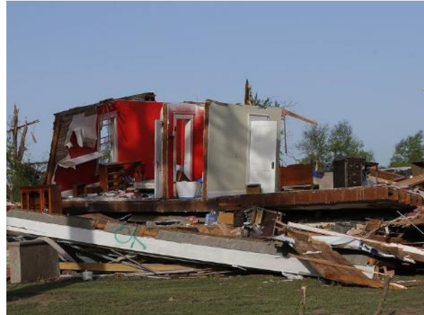
Figure 6. Degree of Damage 7 (113 mph - 153 mph). Possibly an EF2 rating.
