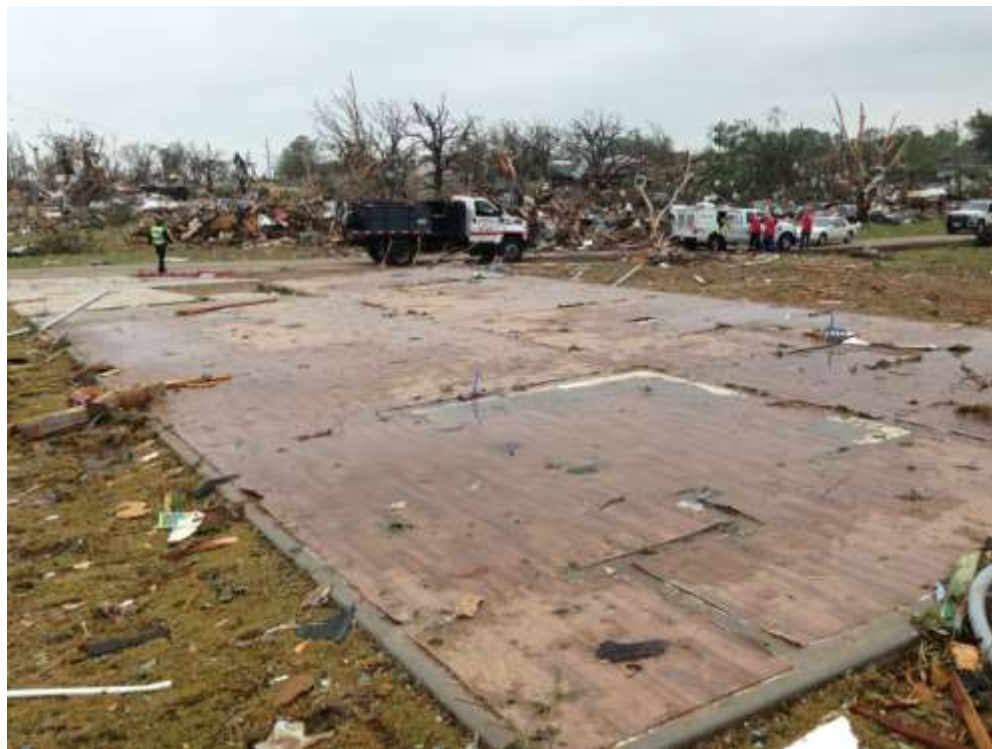
Figure 11: Complete destruction of home just south of Hwy 377 & N. of Acton Highway in Granbury, TX (Image Courtesy of http://www.srh.noaa.gov/fwd/?n=tornadoes051513 )
