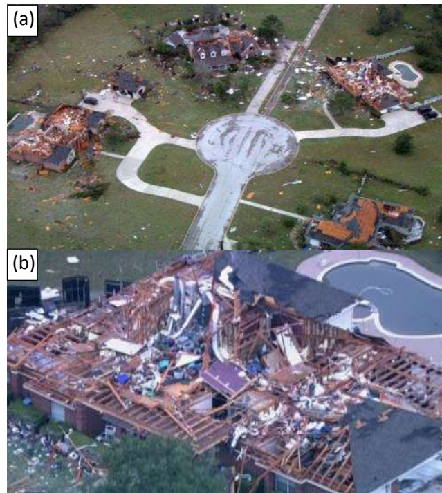
Figure 9: Observed Damage in Cleburne, TX (Credit: WFAA)
